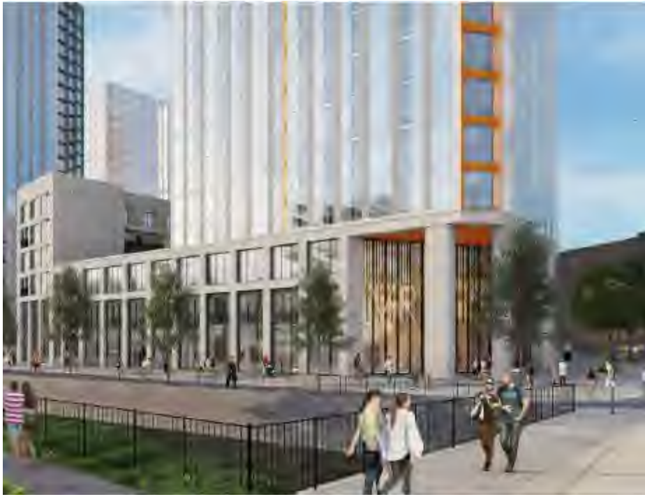
Entrance to tower A and the commercial frontage to podium A fronting Dantzic Street
